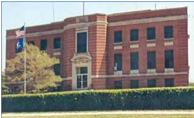
Burke County Courthouse
